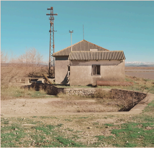
Pumping station: PS 9
